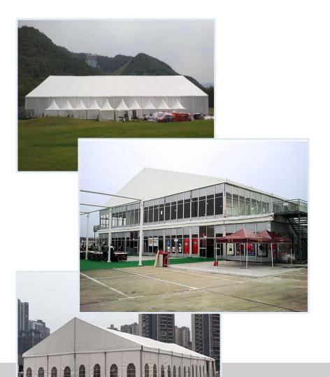
We can offer you the tent as big as 60m span width. The bay distance is 5m, and there is no limits for the length. The big tent is the most widely used tent series for events, weddings, parties, restaurants, commercial, warehouse for permanent usage, exhibitions. Glass walls, glass doors, ABS walls, sandwich walls, air conditioners, flooring, lighting are available.
